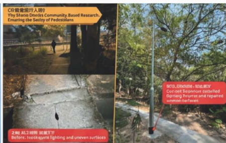
Ensuring Pedestrian Safety: Lighting and Surface Improvements
